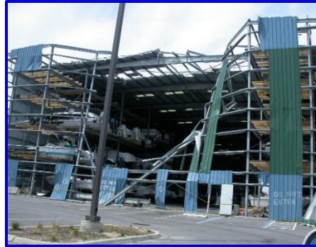
Brooks Bridge Marina
